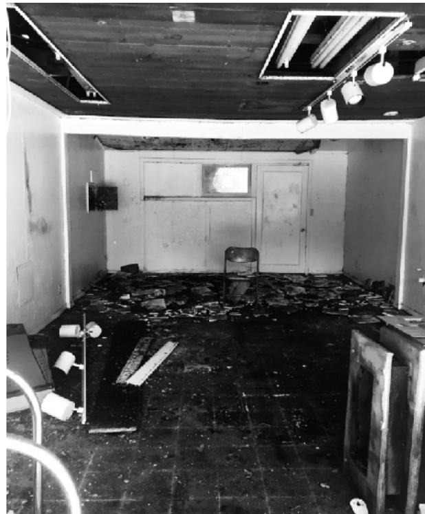
Existing Site Conditions
